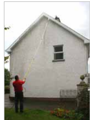
High-reach jet washing for eaves, walls, gutters and downpipes.
